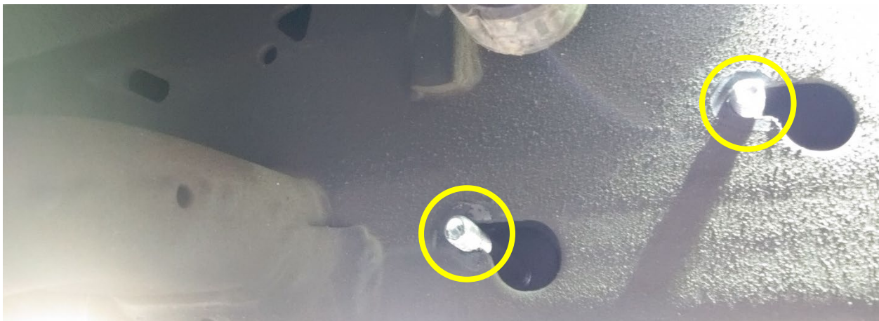
Figure 10- Compressor Bracket Installation, Inside Frame Rail
