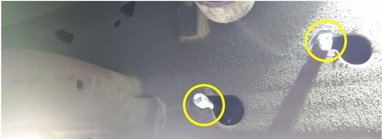
Figure 17- Tank Bracket Installation, Inside Frame Rail
