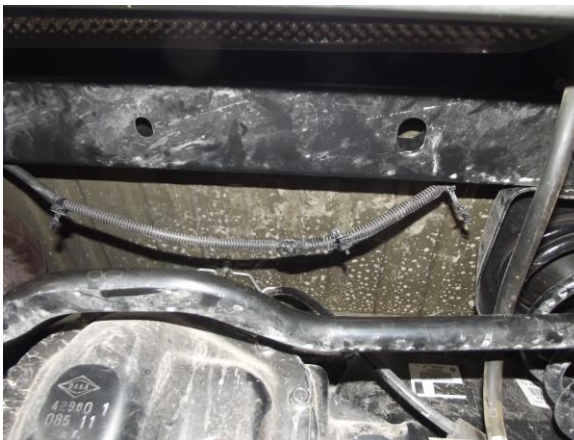
Photo 1 – Horizontal beam with wiring harness clips removed
